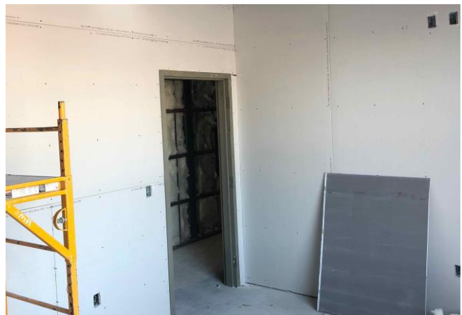
Installed drywall at Office Addition
