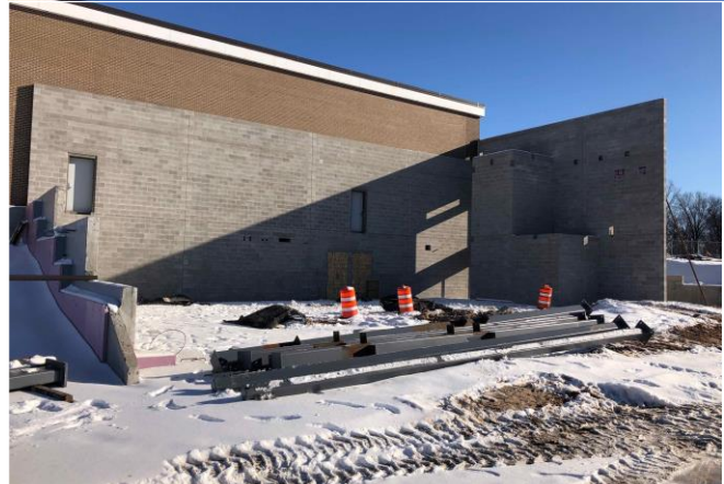
Structural steel delivered for Fitness Addition
