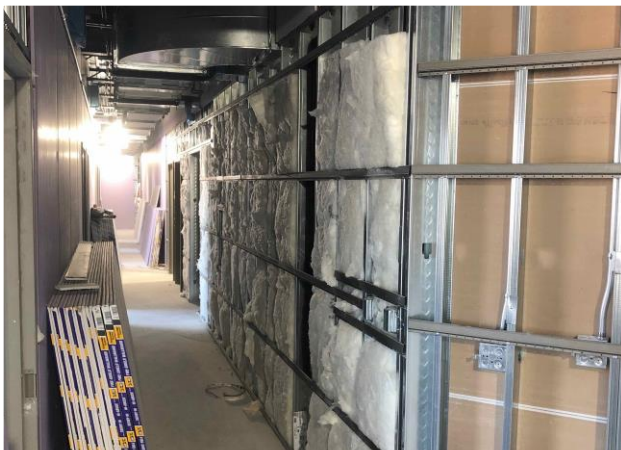
Installed insulation at Office Addition
