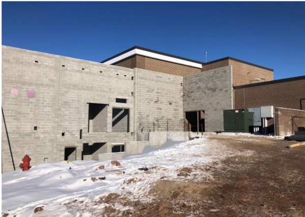
Completed masonry at Fitness Addition
